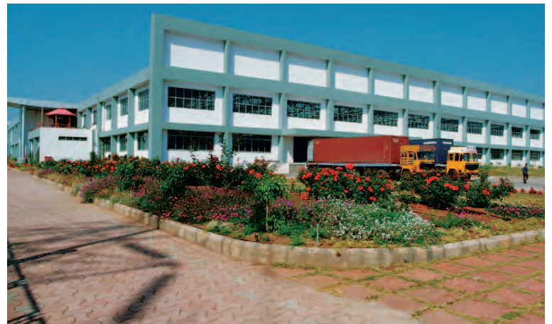
Aluminum Plant Pune, India
