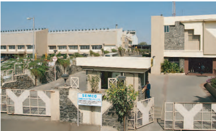
Zinc Plant Pune, India
