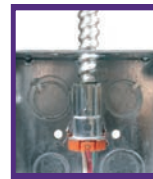
Step 2 Snap conduit into the fitting
