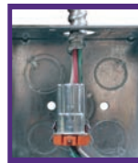
Step 1 Pull conduit thru knockout, insert wires into fitting
