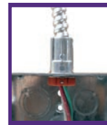
Step 4 Snap into knockout from inside the box
