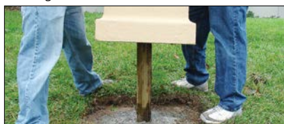
Stucco column ready to install over 4" x 4" post.
