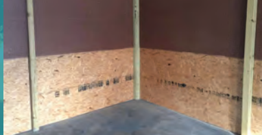
PEG BOARD & OSB INSTALLED
