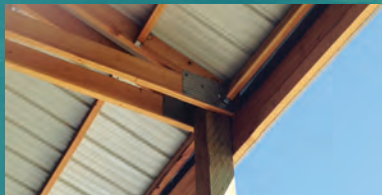
POST TO TRUSS CONNECTION
